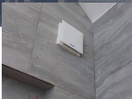
Suitable for less air-tight dwellings, mainly houses, with a design air permeability higher than  $5\text{m}^3 / (\text{h}\cdot\text{m}^2)$  at 50Pa.
